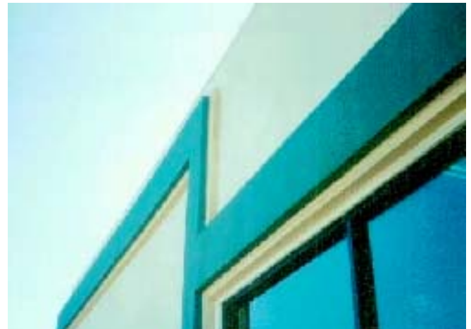
SUPER PLASTER APPLIED TO CONCRETE BLOCK AND INSULATION BOARD BUILD-OUTS
